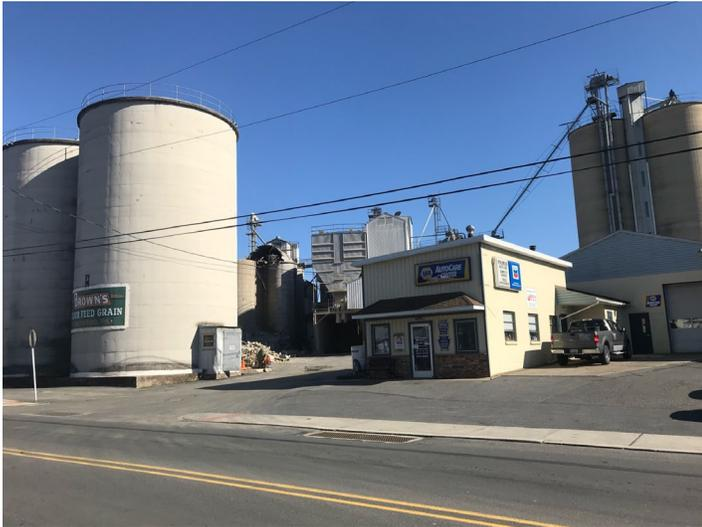
These smaller silos had been built around 1955 and, in the meanwhile, much larger silos had been erected on their property closer to the railroad. Except for the two next to Main St., most of the older silos were 15 ft. in diameter and 50 ft. tall, built in groupings of 4. In contrast, there are 8 newer silos which are 30 ft. in diameter and 100 ft. in height. Behind them are two which are 50 ft. in diameter and 100 ft. high.
